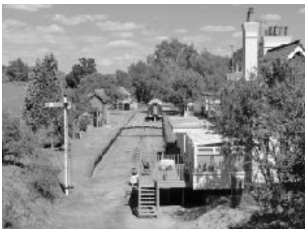
Braughing Station on the Buntingford Line
